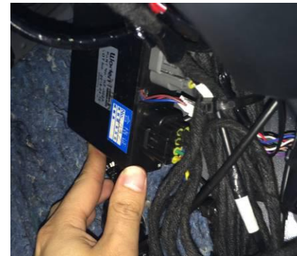
6) ECU fixing position and find negative nearby to connect
