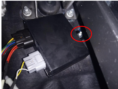
7) fixing ECU as above picture
