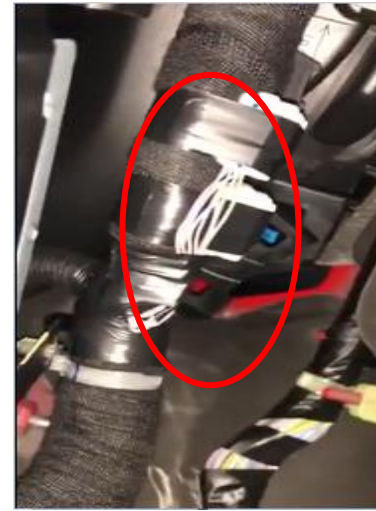
Connector covered by tape along with wiring
